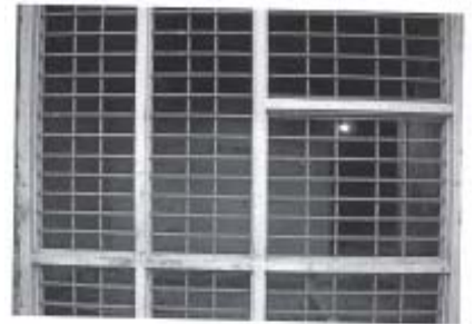
An example of parallel bar design - Horizontal and vertical - with bars passing through wood and going onto the walls
